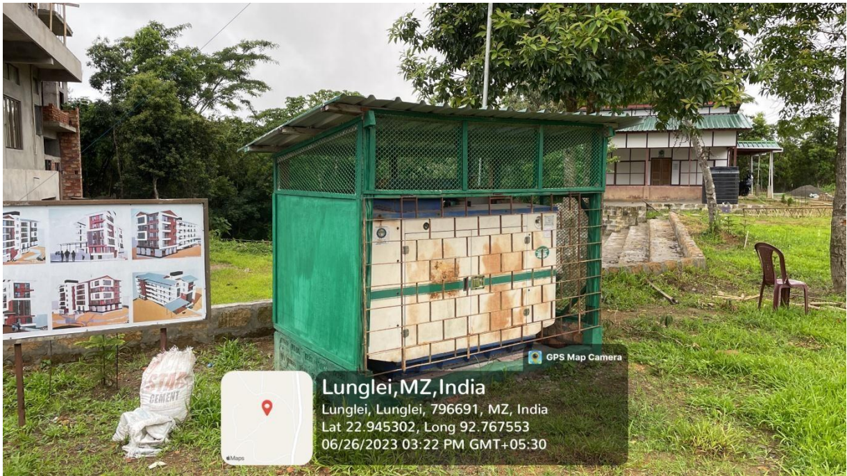
Pic: 10 KVA Kirloskar Diesel Generator
